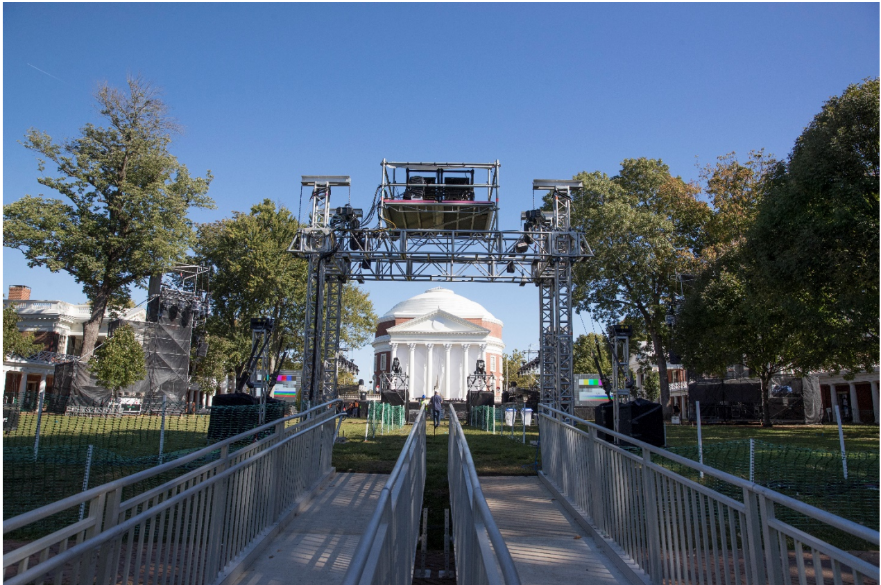
Figure 1: Temporary structures being erected for the University Bicentennial celebration
