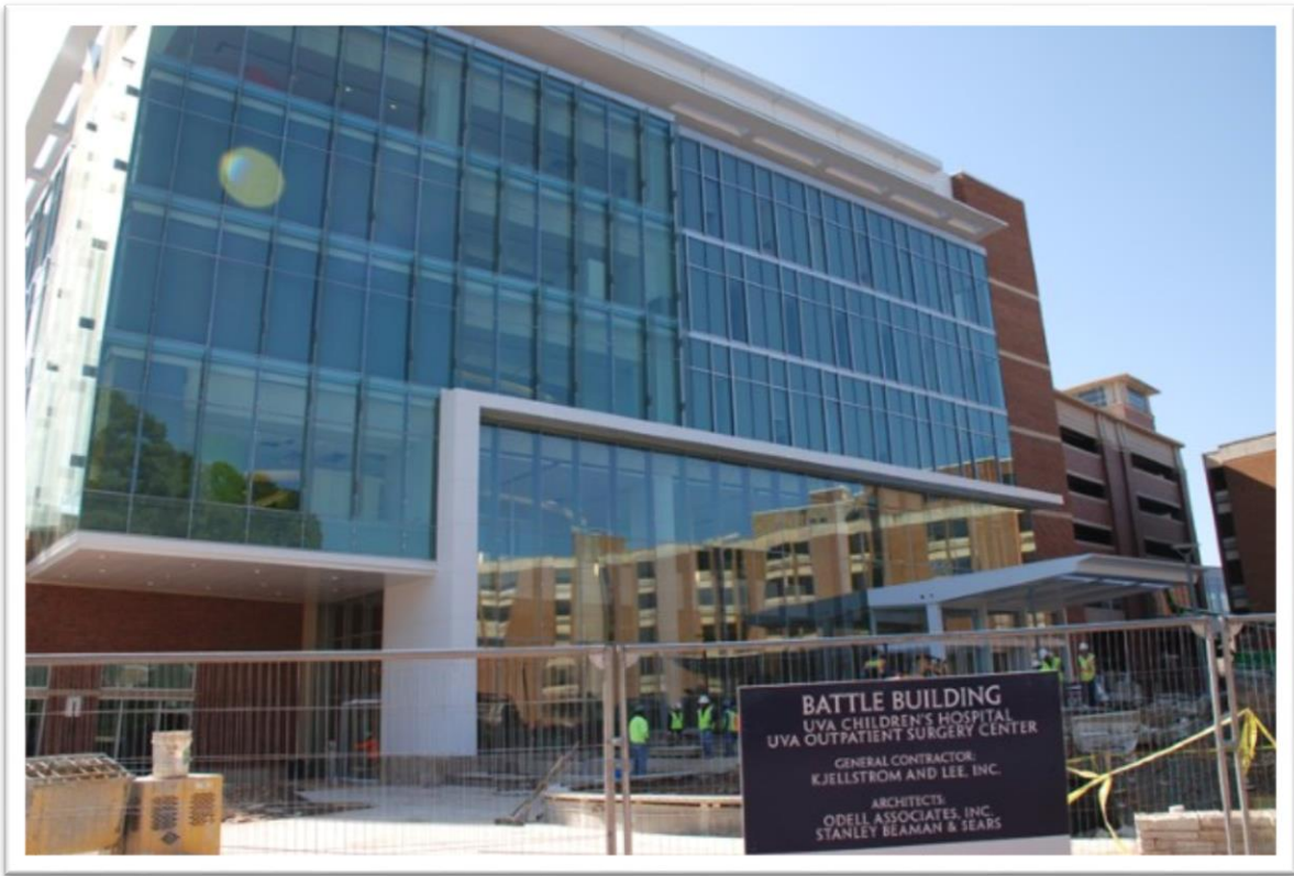
BATTLE BUILDING UNDER CONSTRUCTION
