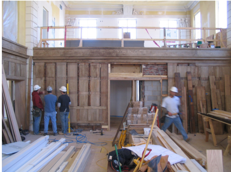
Figure 5 - Garrett Hall Renovation - Occupancy Scheduled July 2011
