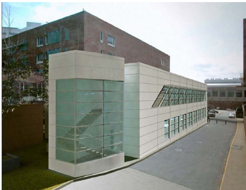
Primary Care Center Annex Occupied February 2010
