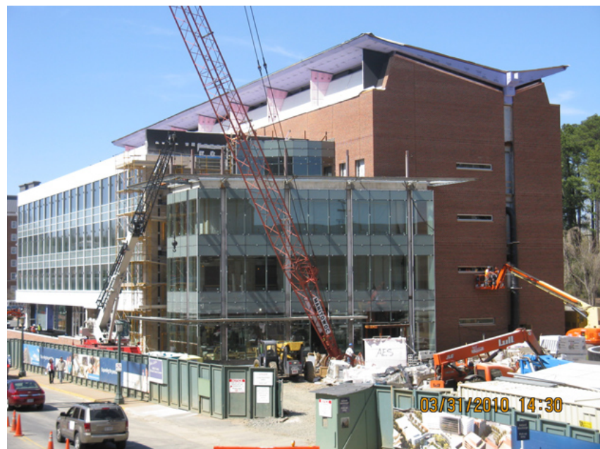
Emily Couric Clinical Cancer Center - Currently Under Construction
