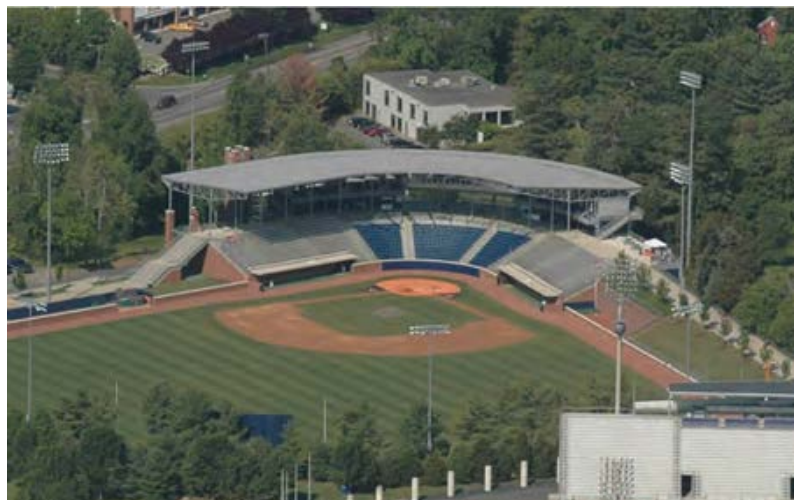
Baseball Expansion and Site of Four Additional Temporary Permits for Increased Spectator Seating - Occupied Spring 2010
