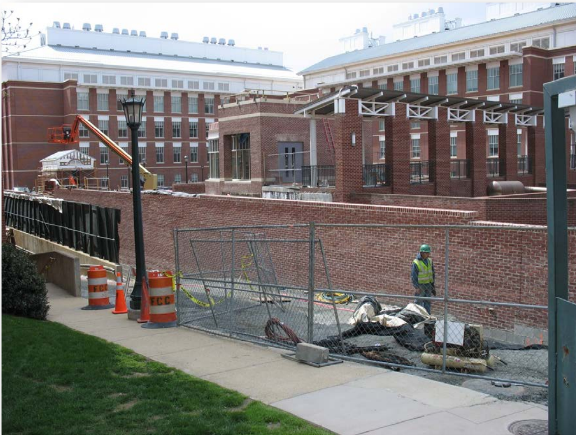
Carter-Harrison Research Building Nearing Completion
